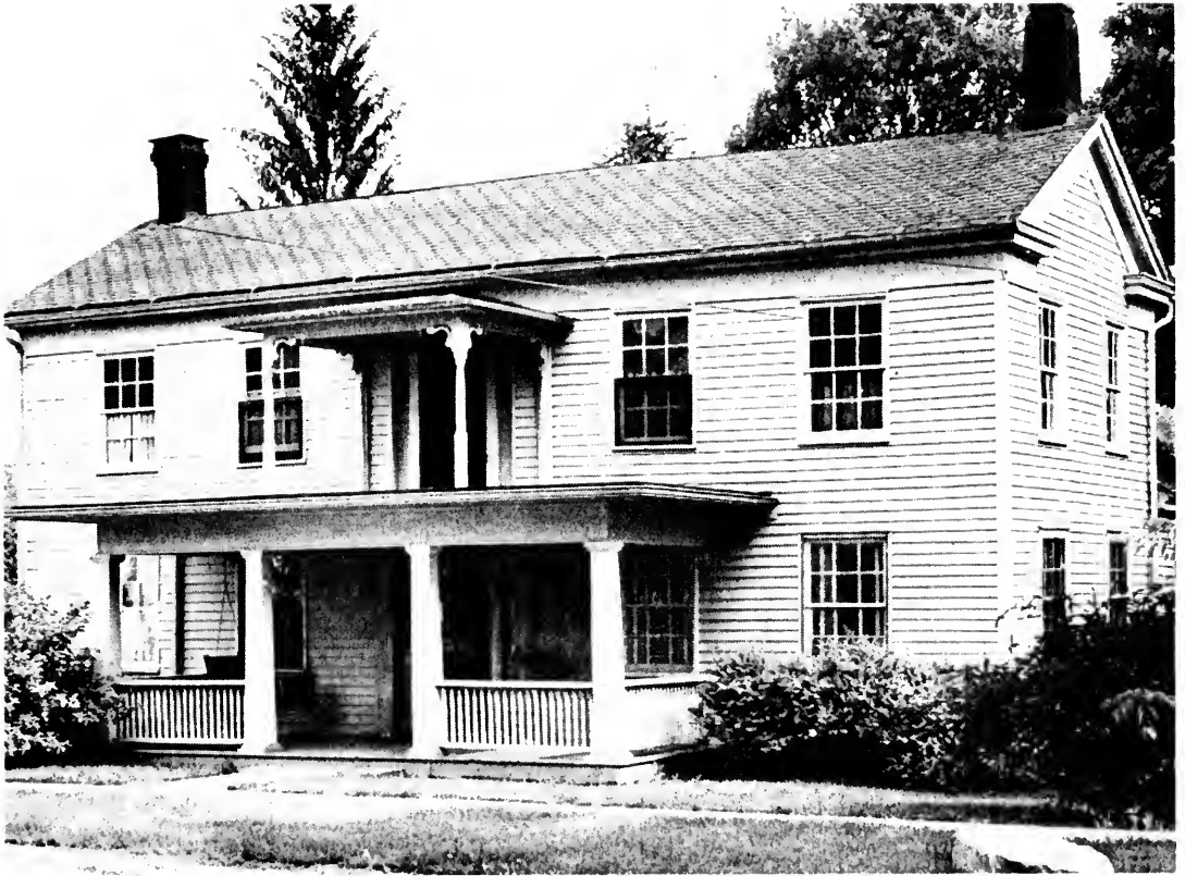
Original Dr. W.B. Noecker home that stood on the East side of the public square
